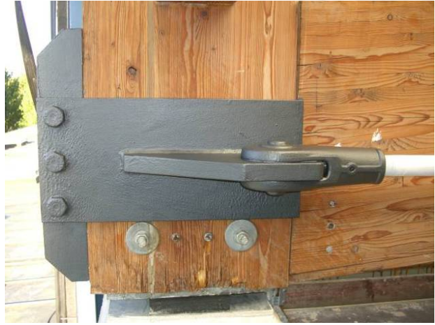
Fig. 22: Connection of the Tensile Bar
