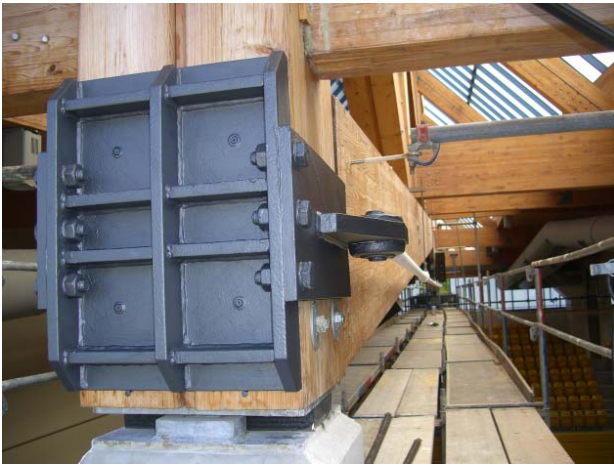
Fig. 21: Pre-stressed steel Tensile Bar
