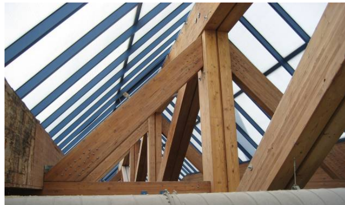
Fig.13: inclined Bar of the Secondary System
