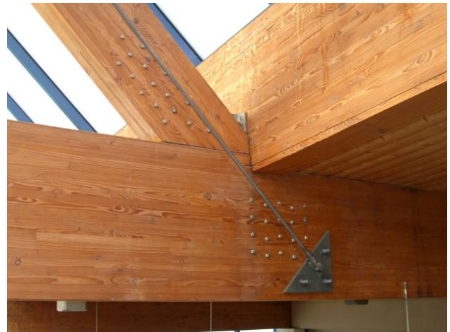
Fig. 20: Connection of the Tensile Bar
