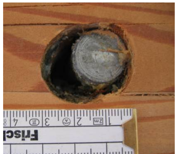
Fig. 4: Indentation of Dowel into Timber
