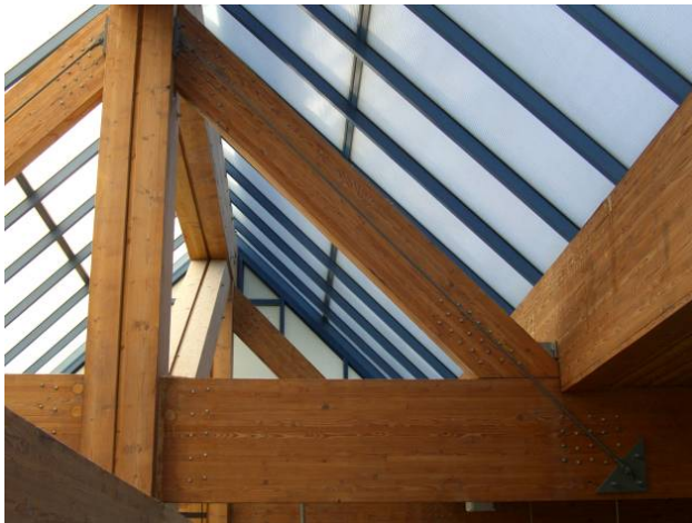
Fig. 19: Pre-stressed steel Tensile Bar
