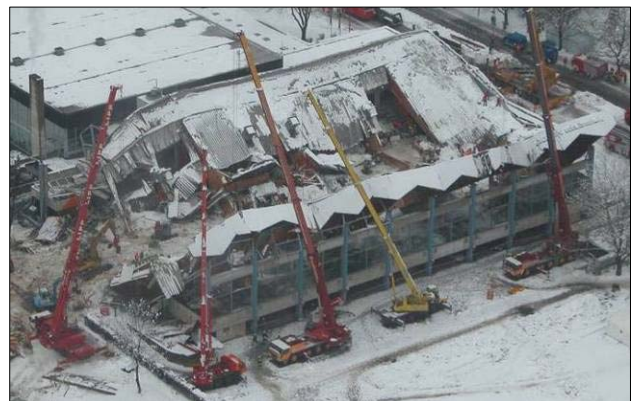
Figure 6: Top view on Bad Reichenhall Ice-Arena after progressive collapse of all main girders [12]
